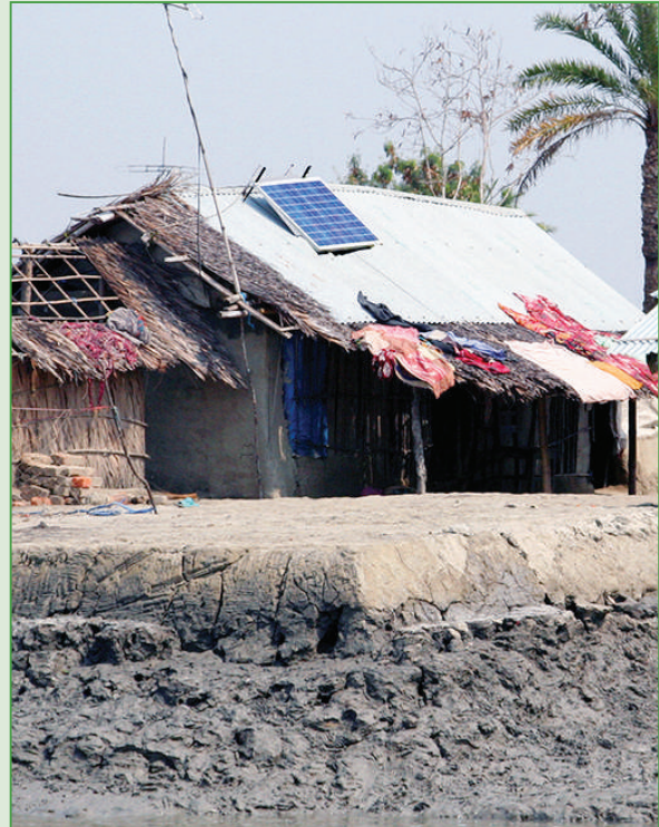
Solar technology is an effective and environmentally sound way to provide most of the people in the rural areas with electricity.
